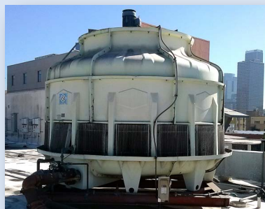
160 ton cooling tower
